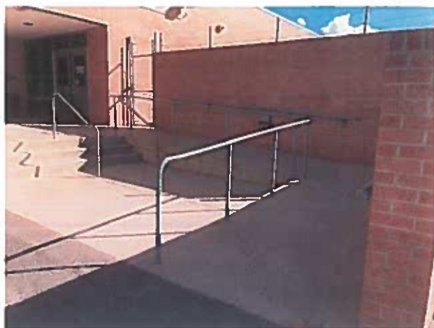
Ramp exceeds 1:12 slope.
